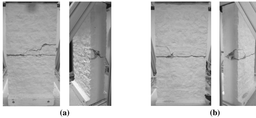
Figure 8. Post-test crack patterns observed on specimen: (a) W4, and (b) W5.
